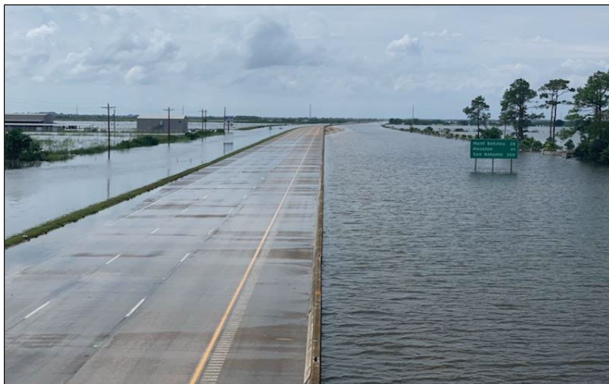
Figure 2 - Imelda Flooding to Median Height
