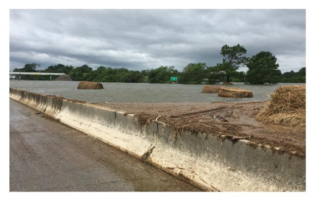
24. Likewise, in September 2019, TxDOT's median barrier/dam along IH-10 blocked rainfall runoff from overtopping the roadway during and after Tropical Storm Imelda. During Imelda eastbound traffic lanes remained open and conferred a benefit to the public at large—and specifically
